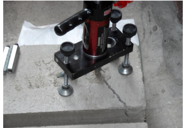
Fig. 10. View of a single sample of concrete cracks during the attempt capacity anchor for pull-out.
