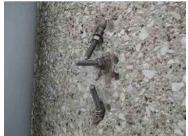
Fig. 6. Anchoring COPY-ECO system and three anchor system.
