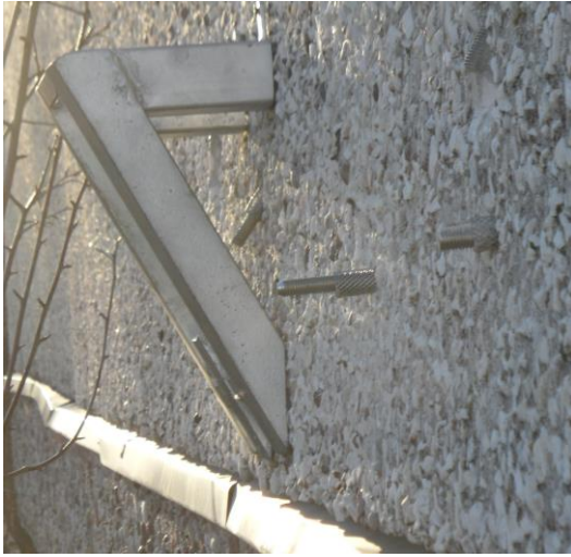
Fig. 4. View of steel frame with anchors.
